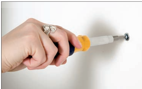
Figure 3-3: Screwing into a drywall anchor for a heavy fixture.
